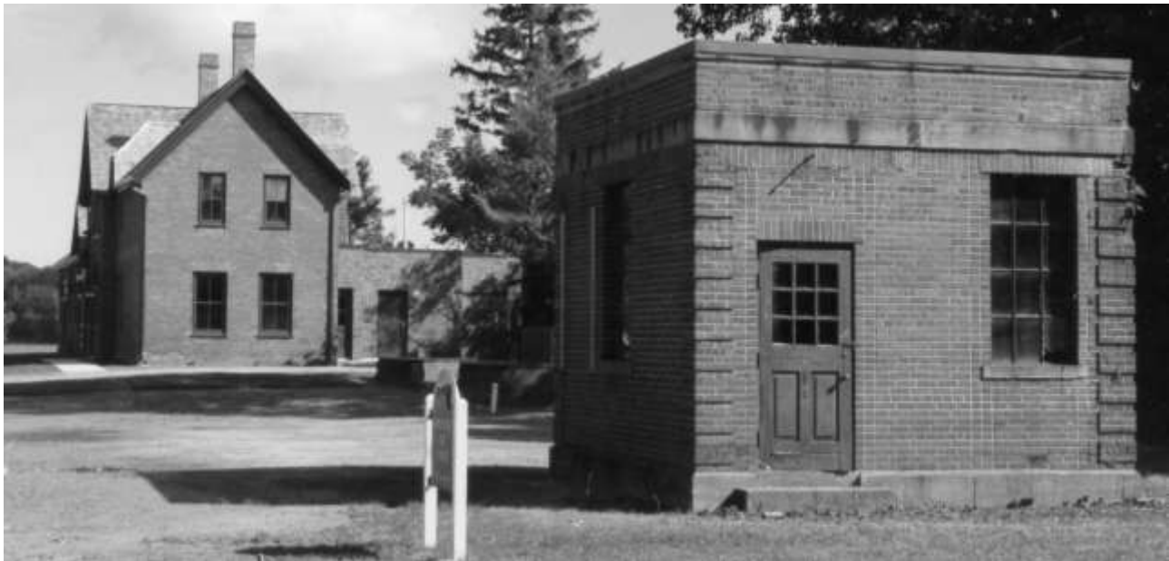
The Niagara-on-the-Lake Waterworks that operated for over 90 years. 1994. The electrical substation is shown in the foreground. [Courtesy: Donald Combe]
