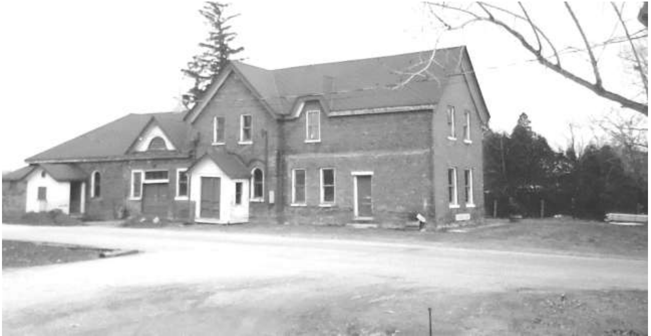
The Pumphouse from the southeast in the 1980s. [Courtesy: Niagara Historical Society & Museum]
