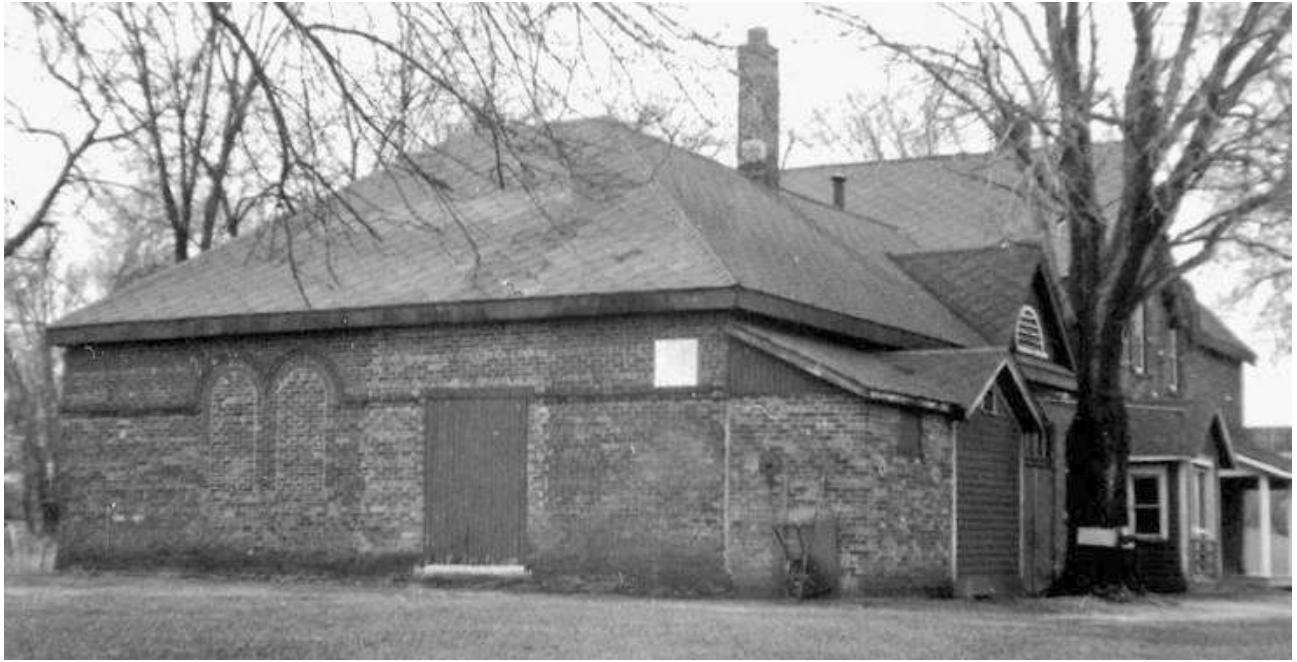
The old waterworks at the Pumphouse in 1957. [Courtesy: Donald Combe]
