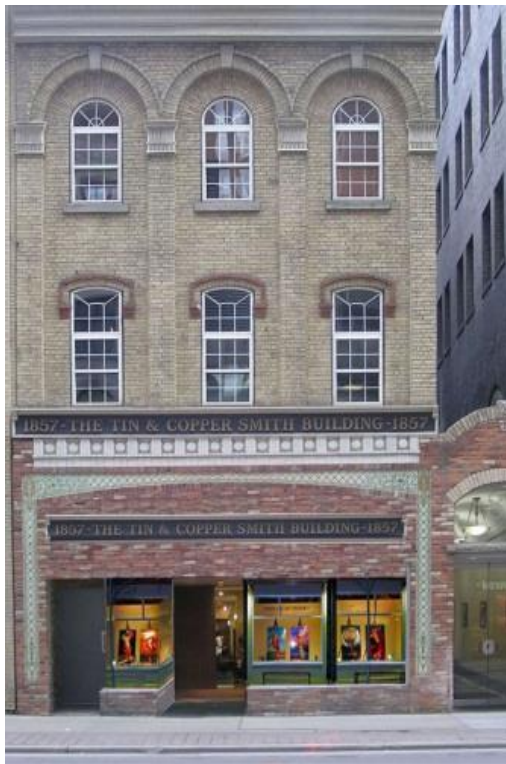
Restored Piper Building- 83 Yonge Street
